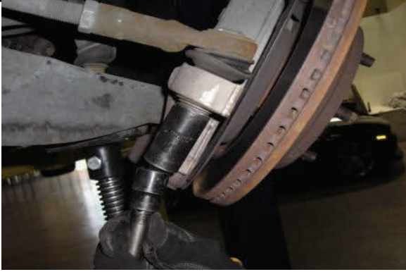
Disconnect tie rod end nut and break loose with hammer
