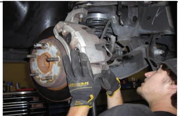
Reconnect brake calipers, sway bar end links, and tie rods.
