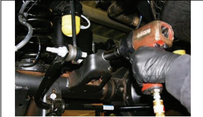
Support rear suspension and remove rear trac bar bolt
