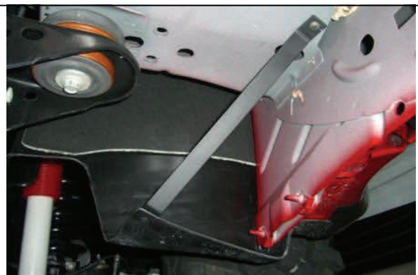
(05-10) Install fender liner strap to clear larger wheel/tires
