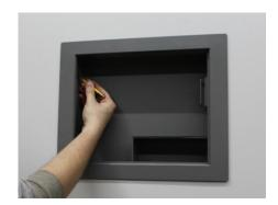
6. Pre-drill 4 pilot holes using a drill and the 1/8" drill bit. Place the wall safe back into the cut out, replace the drill bit with a Philips head bit and secure all four mounting screws into place. Installation is now complete.
