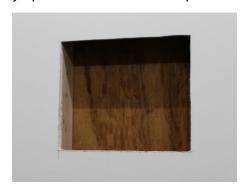
5. Take the wall safe and place it into the square cutout. Make sure for proper fitment and make any adjustments. Open and remove door. Locate the four mounting points. Using a pencil, mark the location for the mounting screws. Mark all four points. Remove the wall safe and place aside.
