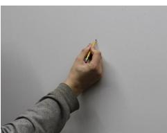
3. Using a carpenter's level draw a horizontal line between these two points. Make sure to maintain a level line. Next Measure down from the end point 12 inches and mark with a pencil. Do the same for both sides. Using the level, draw the vertical lines. Complete the cut-out square by connecting the two bottom points.
